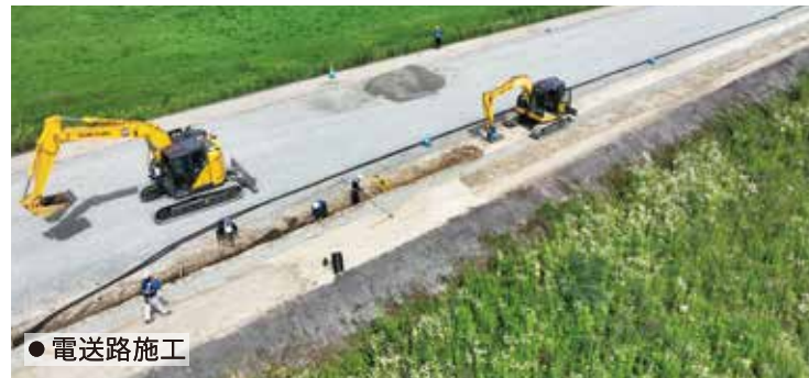
●土砂掘削・積込
